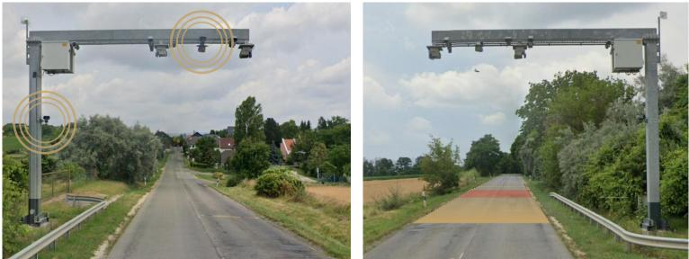
The images above show the test gantry referenced from its two sides. On the left picture (north-northeast view) the two cameras (CAM1 and CAM2) marked with golden rings are facing you. The second image (south-southwest view) illustrates the perspective of the cameras, with the road section highlighted in gold representing the monitored segment. The red highlight marks the Trigger Zone.
